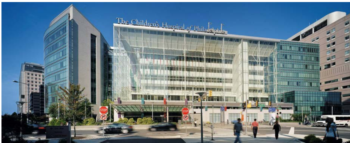
Obr. 1. Nemocnice Children's Hospital of Philadelphia z ulice
